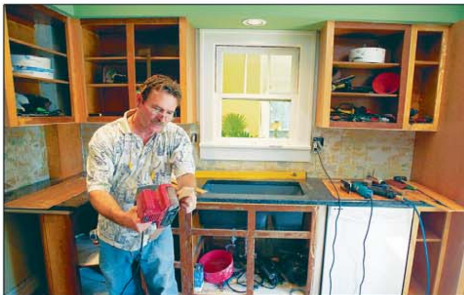
Carpenter Terry Murray uses a sander as he works on refacing kitchen cabinets.
